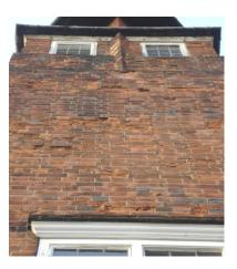
start to let in moisture, which makes the problem worse. Interestingly it seems that this hard mortar was used when the Tower was built, and not during later maintenance - presumably the builders did not expect any problems.
